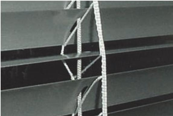
**Image 4** Example of incomplete turning of the slats
